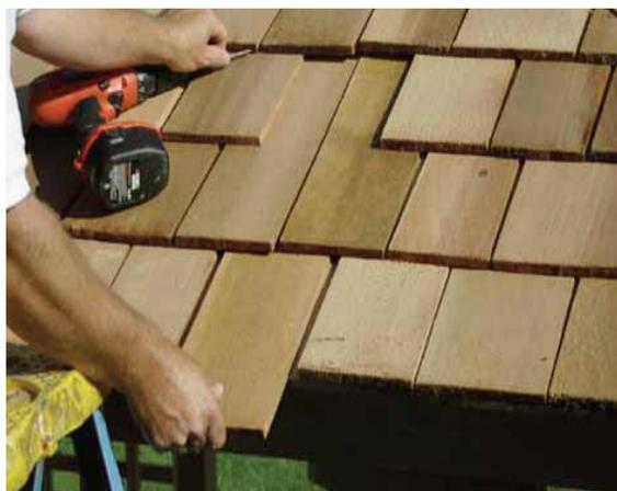
**43.** Roof **Filler Shingles** are included to cover roof seams. Starting at the bottom, slide the first Long Shingle in until flush with other bottom shingles.
