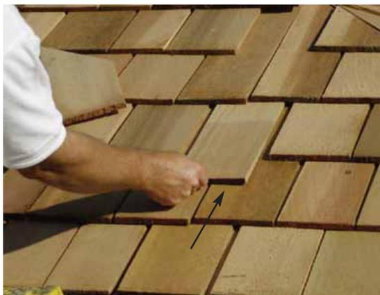
**45.** Slide in another filler shingle and attach as per **Step 44**. On your last row of shingles, attach smaller filler shingle with **2 - 1 1/2" Shingle Nails** near the top, to be covered by Ridge Caps in **Step 60**. Complete all four rows of filler shingles where roof seams meet in the same way.
