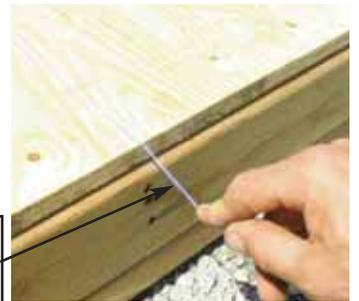
**7.** When completed, make sure the floor is still level and make adjustments if required. When completed, your floor should look similar to this.
